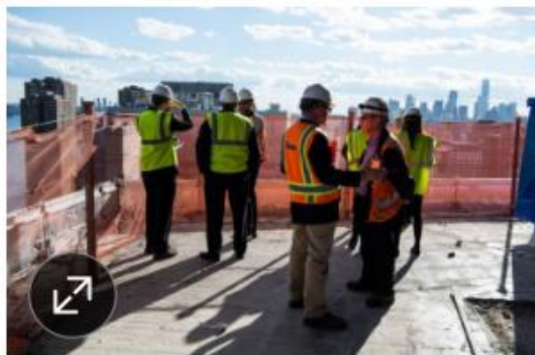
Workers on one of the top floors of an NYU Langone construction project in October. PHOTO: MARK KAUZLARICH FOR THE WALL STREET JOURNAL
